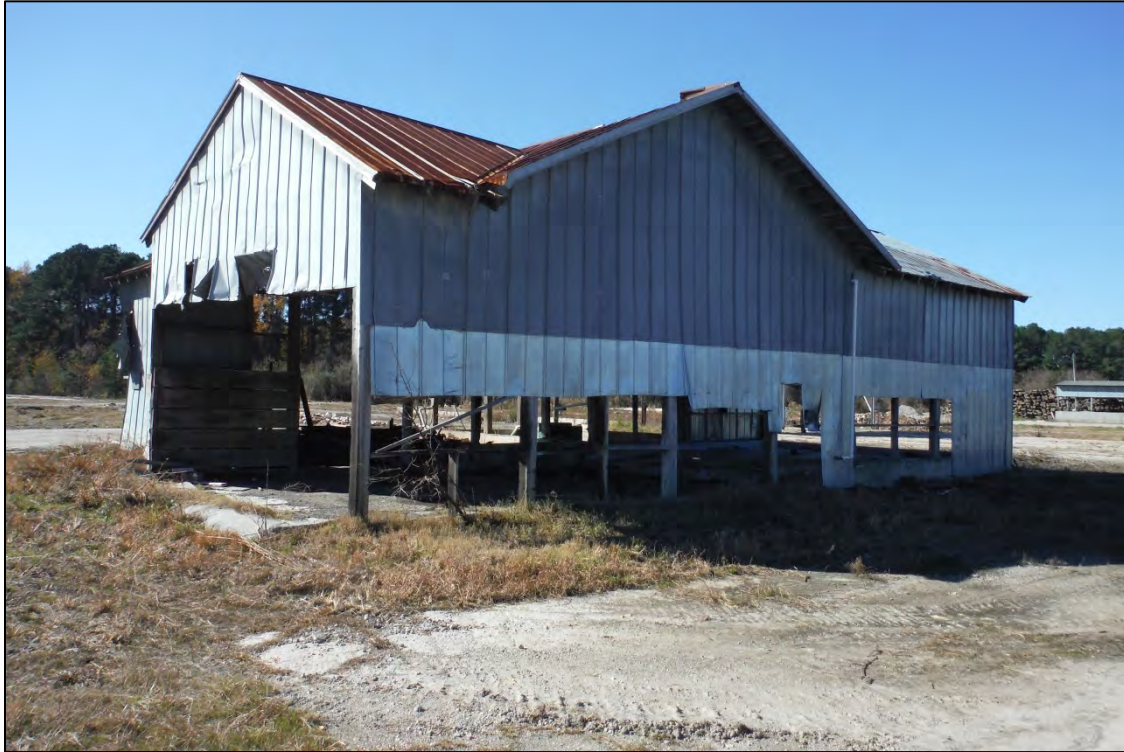
Figure 10. HX1598, Structure 5, facing northeast.
