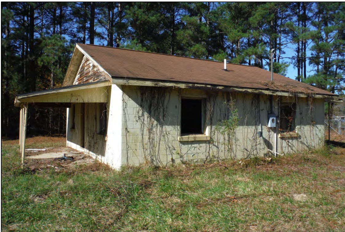
Figure 9. HX1598, Structure 4, facing northwest.
