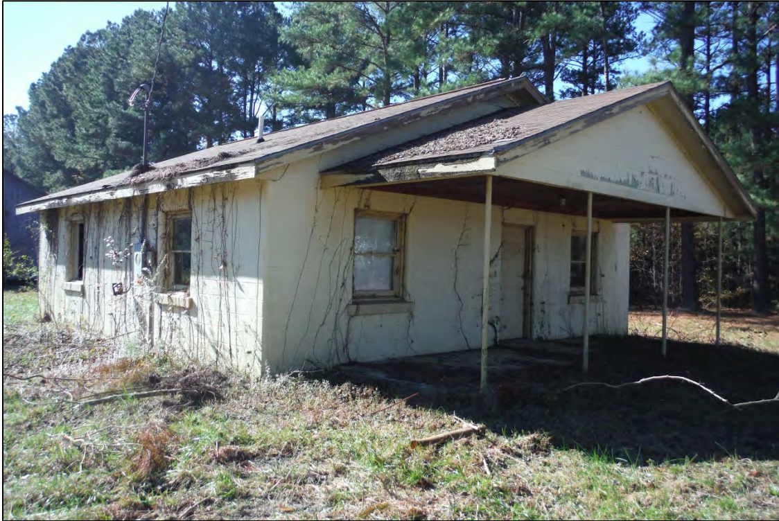
Figure 8. HX1598, Structure 4, facing southwest.
