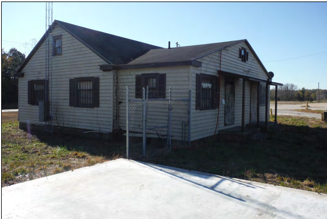
Figure 5. HX1598, Structure 1, facing southeast.
