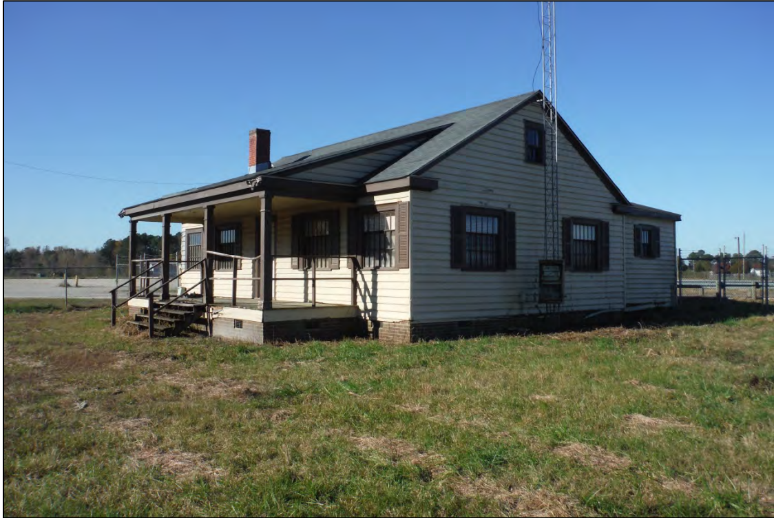
Figure 4. HX1598, Structure 1, facing southwest.
