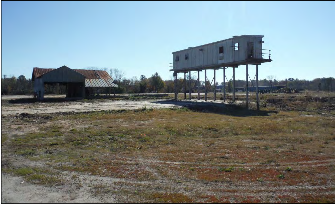
Figure 12. HX1598, Structure 7, facing east.
